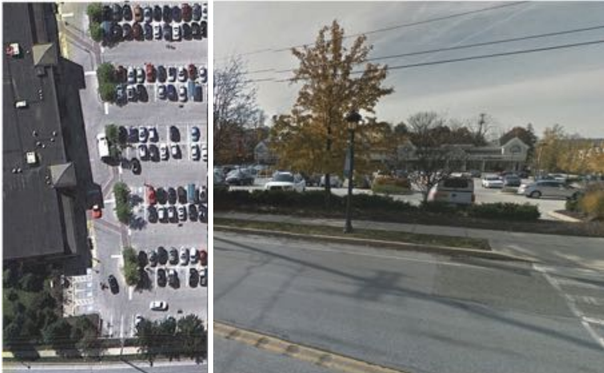
Paoli Shopping Center in Chester County. Note the internal and external crosswalks, sidewalk, greenspace, and the tree wall that faces the road.
