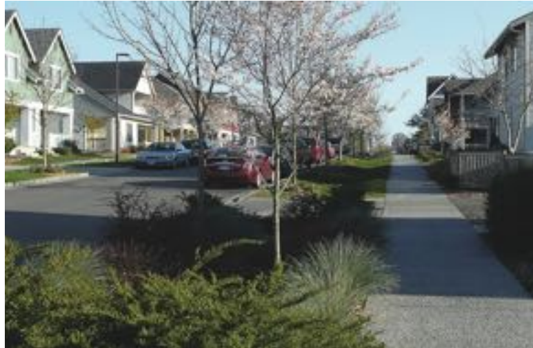
Residential rain garden and strip with bioswales and rain gardens next to permeable sidewalks (below). These examples of “green infrastructure” can be employed in residential areas to control stormwater runoff, and decrease the impact on local streams.
